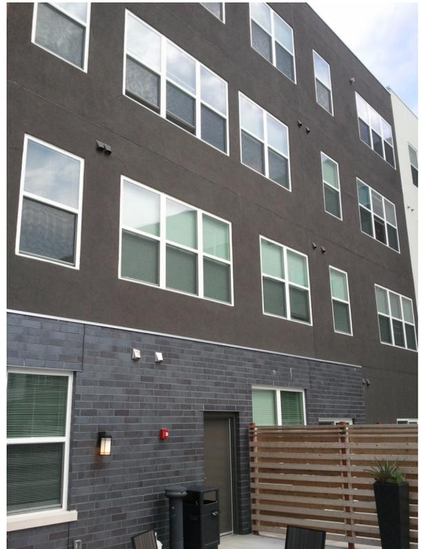
This black building melted the insulation board shortly after installation. White and gray panels on either side were fine. Avoid large, dark surfaces with EIFS.
