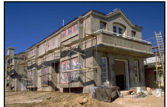
Finishes dry differently in the shadows of the scaffolding
