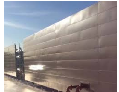
Example of oil canning a.k.a. buckling or surface variation on a metal building
