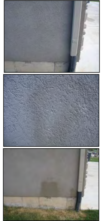
Top: Test Wall Middle: Muriatic acid fizzes on wall Bottom: Dried and restored finish
