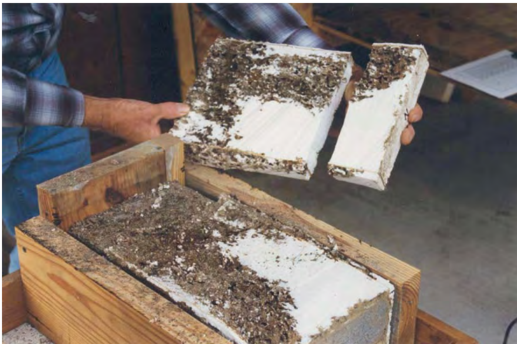
#45 TEST FIXTURE - cut open to reveal extensive termite damage.
