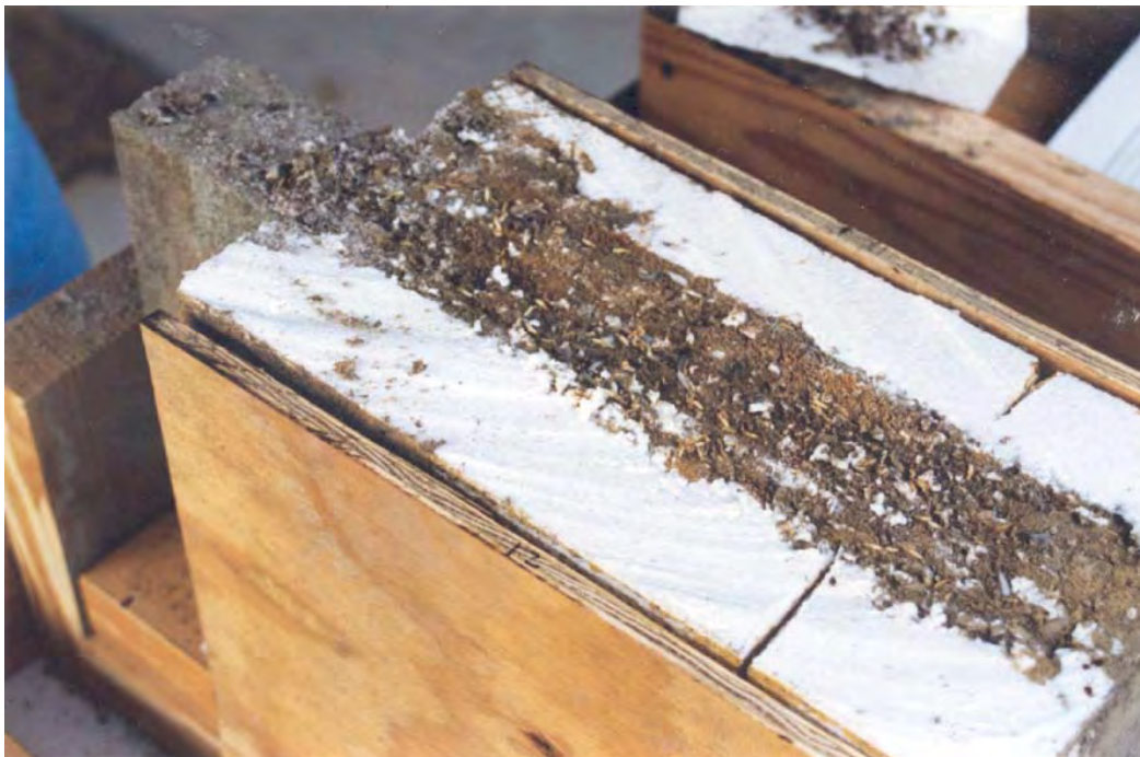
#45 TEST FIXTURE - Close-up shows active termites.
