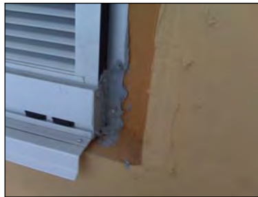
Rollershield along with Rollershield Flashing Tape easily conforms to wall irregularities.
