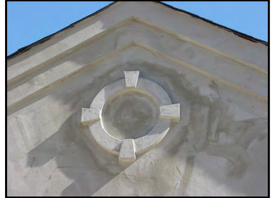
Stucco with Foam Trim (Not EIFS)
