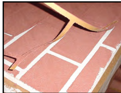
Remove Stencil as brick color is setting up
